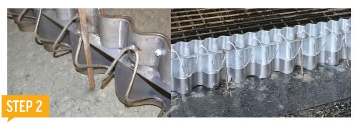
Hammer or drill pins (max. Ø 16 mm?) into the ground vertically (slightly inclined in the direction of the joint longitudinal axis) inside the anchorage system with 2 on each side at the end of the profile. At least 2 additional should be attached approximately in the middle of the profile (1 on each side) to ensure the correct position of the profile and to enable necessary adjustments.
