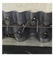
Check again the height level of the profile at the beginning, the middle and the end with a laser and also the horizontal and vertical level. Weld the pins to the profile. If welding work is not permitted on site, special adjustment feet are available. Pull down the falling steel plate to adjust the joint to the floor slab height.
