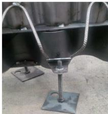
Check again the height level of the profile at the beginning, the middle and the end with a laser and also the horizontal and vertical level. Weld the pins to the profile. If welding work is not permitted on site, special adjustment feet are available.
