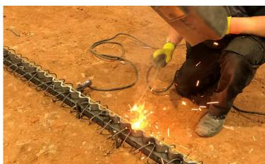
Place the next profile with its overlap of the sinus wave on the first profile. With the overlap, the start of this profile is immediately at the correct height. Bring the middle and the end of the second profile to the correct height with laser and weld first the upper waves of the two joints. Repeat step 3 and 4 and weld the profiles together. Continue this way until arriving at an intersection, wall or column.
