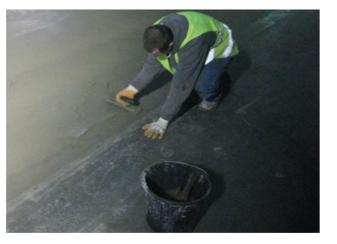
Compact the concrete with needle vibrators in order that trapped air and excess water are released and the concrete settles firmly along in the joint. Avoid polishing the concrete over the joint. To become a satisfied result of the sinus slide® jointing solution, it is absolutely necessary to finish carefully the concrete at the same level as the sinus joint edges. SEE BACK SIDE OF THIS GUIDELINE.
