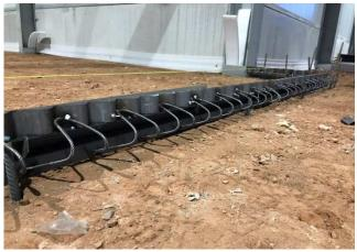
Hammer or drill pins (max. Ø 16 mm) into the ground vertically (slightly inclined in the direction of the joint longitudinal axis) inside the anchorage system with 2 on each side at the end of the profile. Two additional pins should be attached approximately in the middle of the profile (1 on each side) to ensure the correct position of the profile and to enable necessary adjustments.
