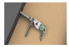
Then drill and fix deformed bars ( $\emptyset 16 \times 600$  length) in each concrete slab. At least 3 dowels per meter in each concrete slab. 300 mm of the dowel must be fixed in the concrete (ideally with resin anchorage system) and 300 mm must stick out. Apply special primer on all vertical sides of the concrete slab.
